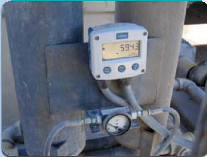
Bearing Temperature Monitoring on a Ferry
